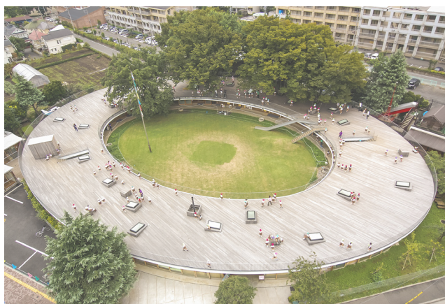
Fuji kindergarten - Tezuka architects, Tokyo
