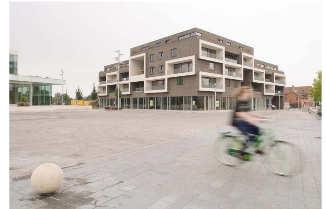
Hertogloges | Lommel BE Team: plusoffice architects
